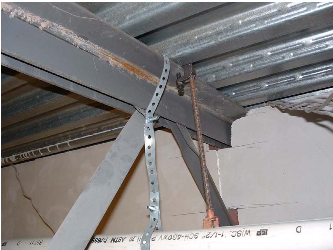
Fig. 7 Joist with Crimped Web Members.
