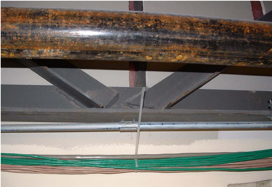
Fig. 14 Web Angles on Side of Chords
