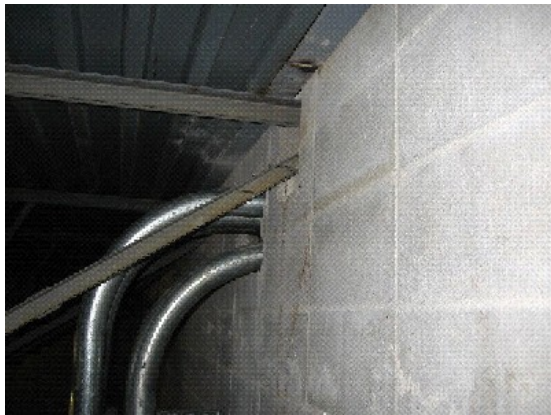
Figure 1 Joist End Diagonal Webs Inadvertently Cut During Construction
