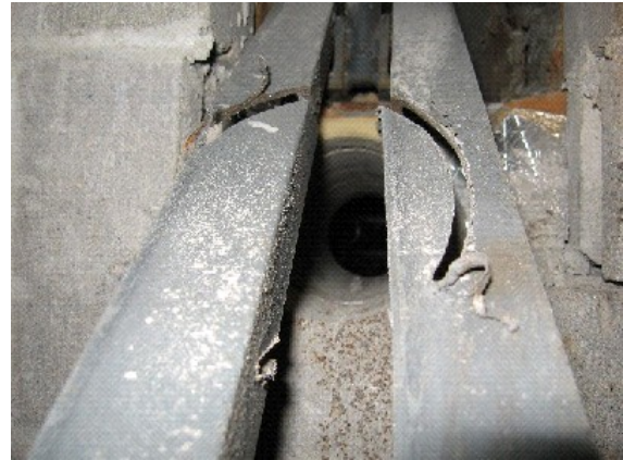
Figure 1 Joist End Diagonal Webs Inadvertently Cut During Construction
