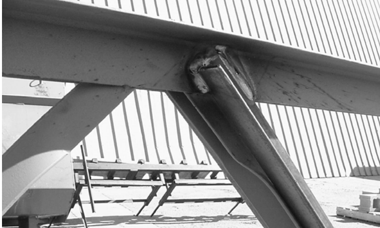
Angle Reinforcement on Crimped Web Joist
