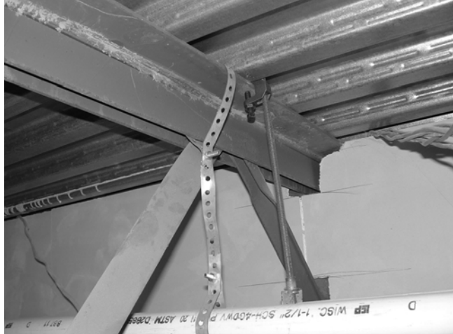
Joist with Crimped Web Members
